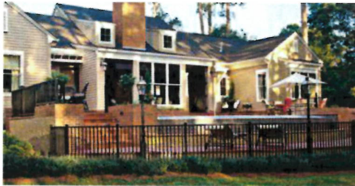
Ornate Black Aluminum or Metal 'Picket Fence' 3'-6" Maximum Height Fence Posts not to exceed 4'-0" Maximum Height (front and rear zones, where allowed, see diagram A)
